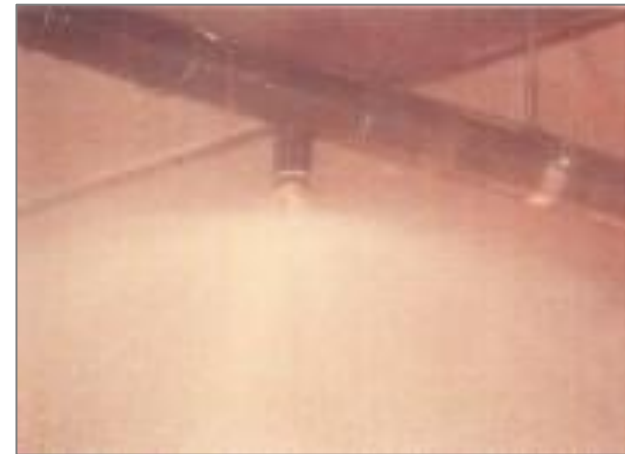
Sprinkler nozzle opens
