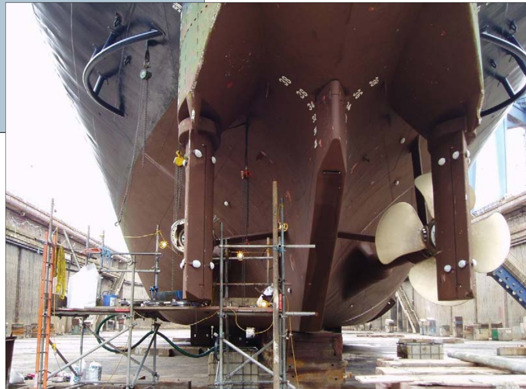
Vessel's stern end arrangement with port propeller blades removed
