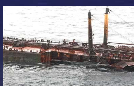
Structural Failure Prestige 2002
